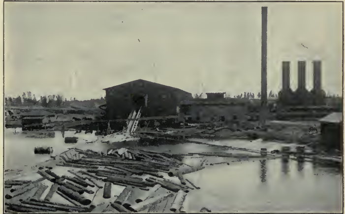
FIG. 250. — A sawmill in Wisconsin. The logs are floated from the forest by the river, and sawed into lumber in the mill.
